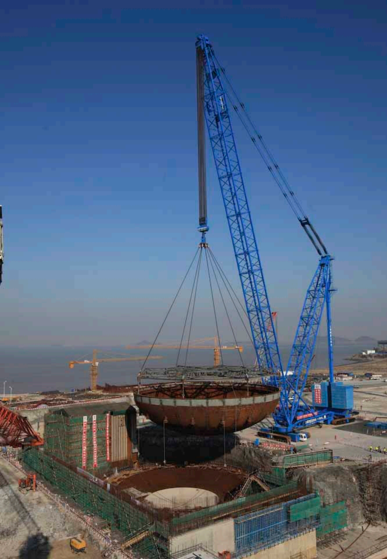
Sanmen Unit 1 - CVBH Lift
