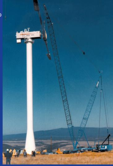
The Lampson LTL-350 and 500 Transi-Lift<sup>®</sup> Mobile Cranes are two models of the World's most versatile Heavy Lift System. These models combine the heavy lift capabilities of Ringer<sup>®</sup> equipped cranes with the mobility of conventional crawler mounted equipment.
